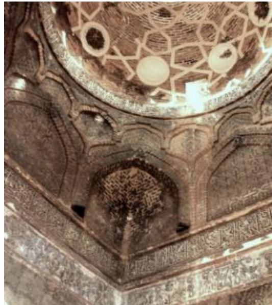
Fig.4. Left: The permanency of the Seljuk pattern of transition zones influenced by architectural achievements in nezamolmolk dome, in the small dimensions of dome. Right: Dome of Jameh Mosque of Qerveh (Photo by Hojat Golchin). Left: Dome of Imamzadeh Aqil in Yasukand Village of Bijar. Photo by: Isa Esfanjari.
