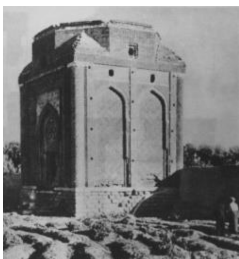
Fig. 5a (Up): The zone of transition of Gonbad-e sorkh and the form of its squinches, a view from inside. Photos by: Hojat Golchin. 5b (Middle) : The exterior of the Gonbad-e sorkh and its zone of transition in the form of an eight-sided prism based on the cube-shaped dome chamber. Photo by Andrade Godard. Source: Godard, 2008: 287.
