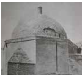
Dome of the Jami Mosque of Qazvin (Godard, 2008, 4: 24)
