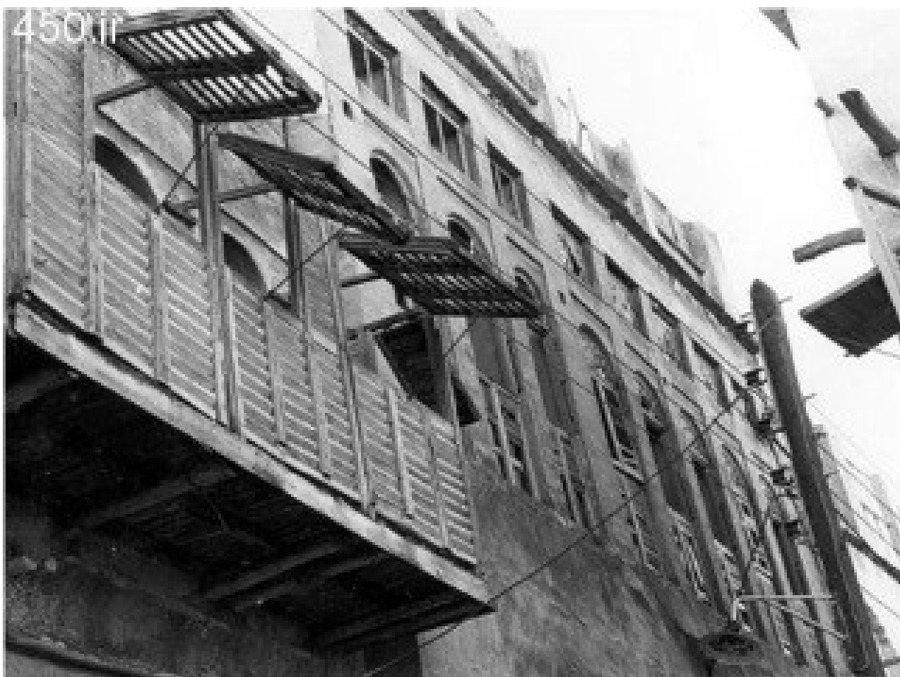
Fig. 5. Structure for creating security and confidentiality. Source: The documents of center of the cultural heritage of Bushehr province.
