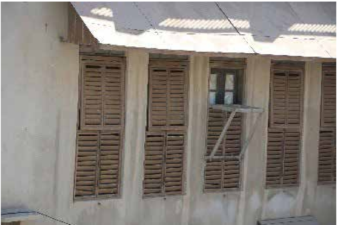
Fig. 4. Similarity of the structure of Senasirs and awning windows without Senasir in front of them. Photo: Bahrani. 2016.
