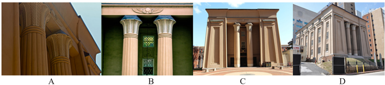
Fig. 2. General form and some details of the medical college in Richmond. A: The shape of the columns and the capitals. B: The prominent shape above the building (winged solar cornice). C: View of pylon towers with an upward slope. Source: www.architectureinrichmond.com. D: Solid form and pure geometric structure. Source: www.roadarch.com.
