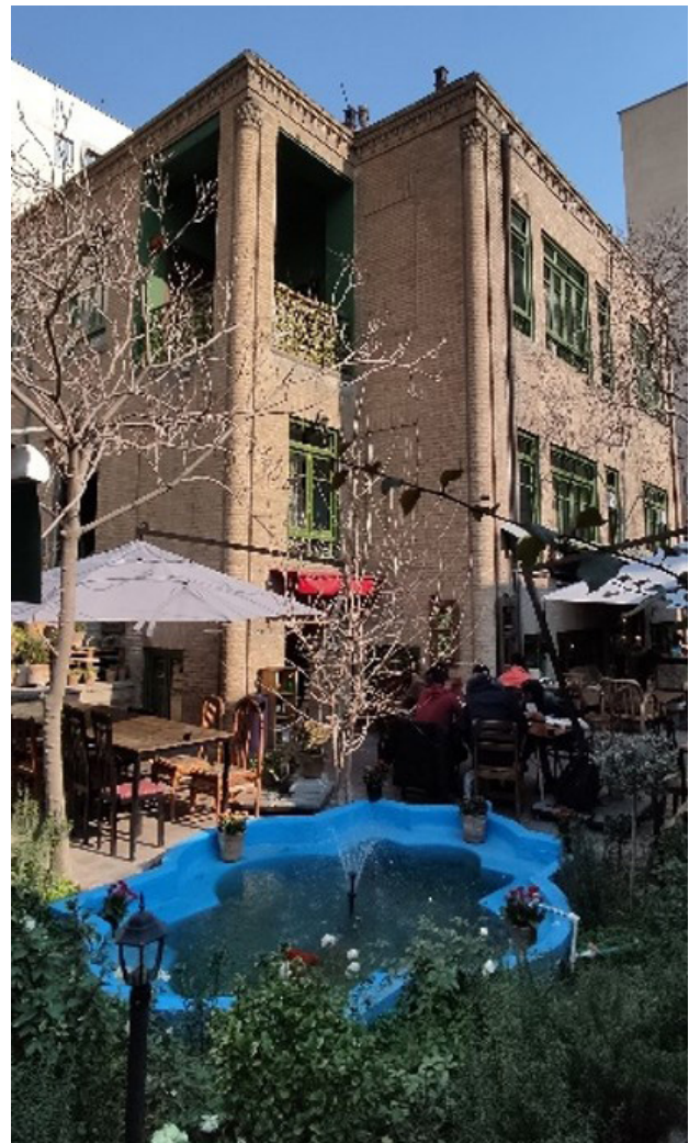
Fig. 33. Overall view of the House No. 3. Source: Authors archive.
