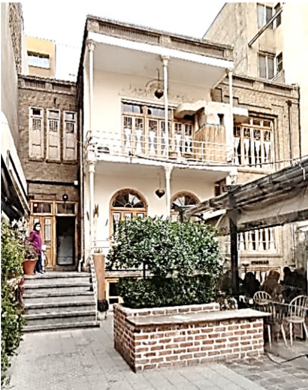
Fig. 8. Overall view of the house No. 2. Source: Authors archive.
