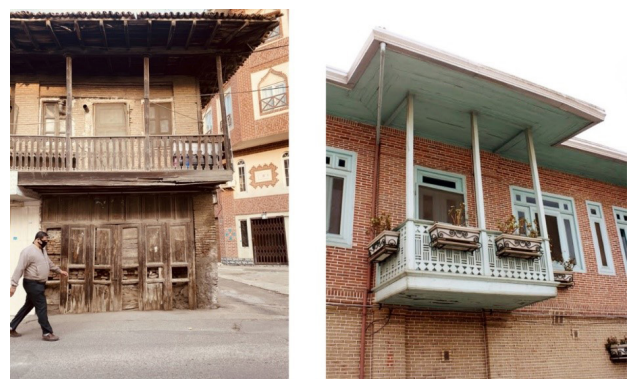
Fig. 12. A projecting terrace facing the alley in houses belonging to the mid and late Qajar period in Babol. Photo: Authors archive.
