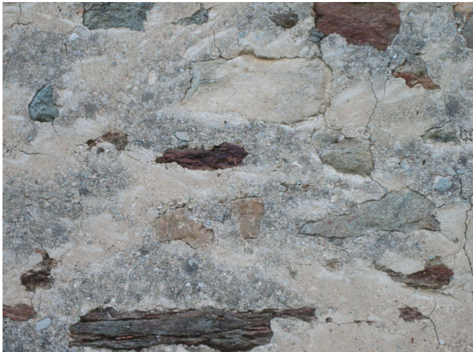
Fig. 7. The Roman technique of Pietra-Rasa plastering. Source: Flüge, 2012; Weyer et al. 2015.
