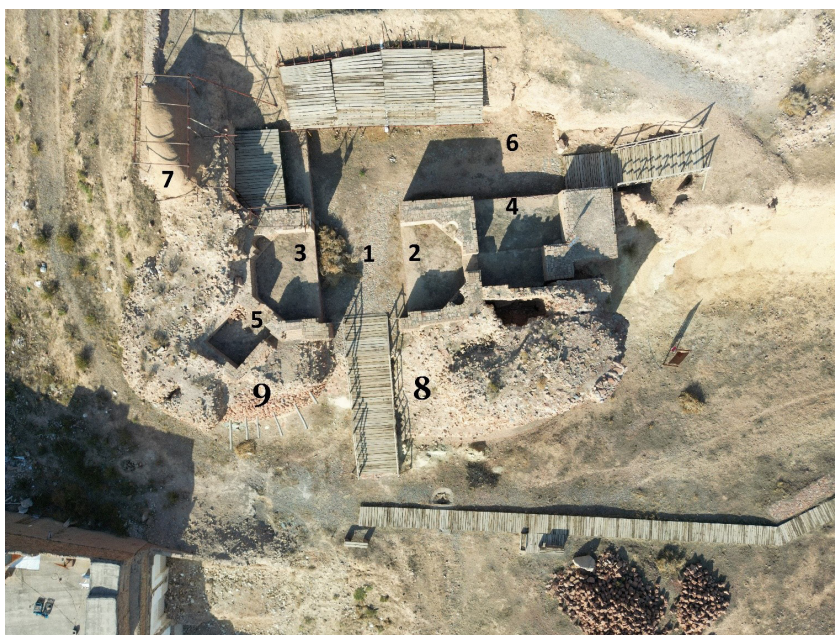
Fig. 4. A drone image (90°) of the SW gate of Rashidiyya: 1. Gate, 2 & 3. Guardhouses, 4. Right back chamber/ embrasure, 5. Left back chamber/ embrasure, 6. Corridor, 7. Remains of the clay wall from the quick repairs by the Safavid Shah Abbas, 8 & 9. Bastions. Source: Ajourloo, 2025.
