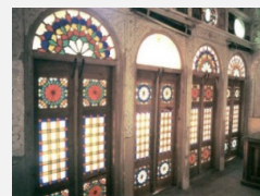
Use of Gereh Chini windows with stained glass in the Lariha House (Qajar Period)
