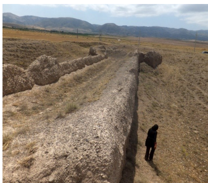
Fig. 15. One of the brick towers of Kalfir castle. Photo: Reza Salmanpour, 2016.
